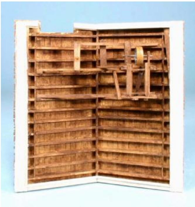
Left: A removable roof was built by Dave Armitage which included the idler pulley. This idler pulley is still in the Power House today (2011). By the position of this pulley and the stack location, it appears the boiler was in the north east corner of the building and the steam engine and drive system in the northwest corner.
