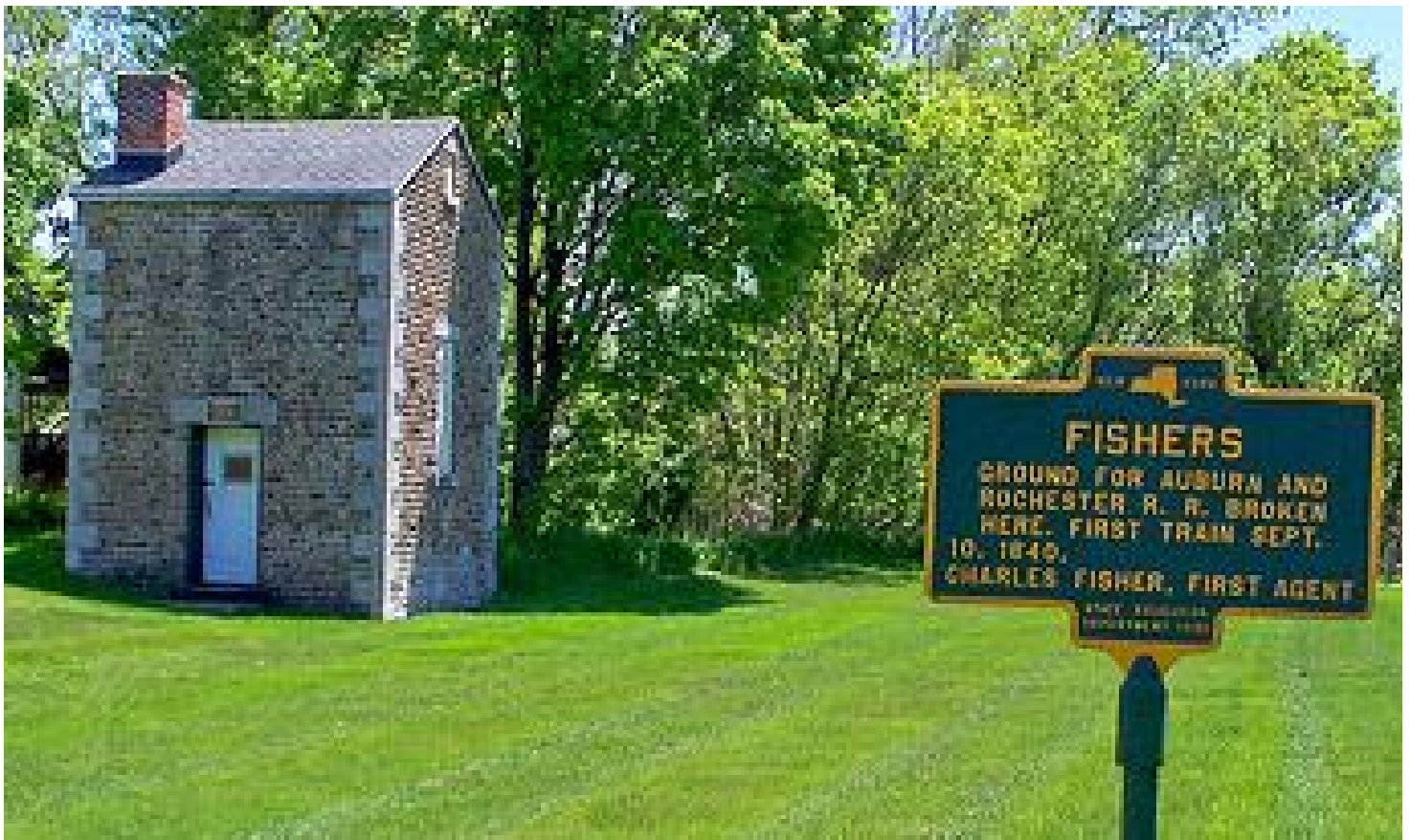
Below: The Stone Pump House in Fishers, NY today – 2012. Sign says FISHERS – Ground for Auburn and Rochester R. R. broken here. First train Sept. 10, 1840. Charles Fisher, first Agent.
